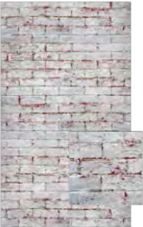
Brick Wall, Peeling Paint
