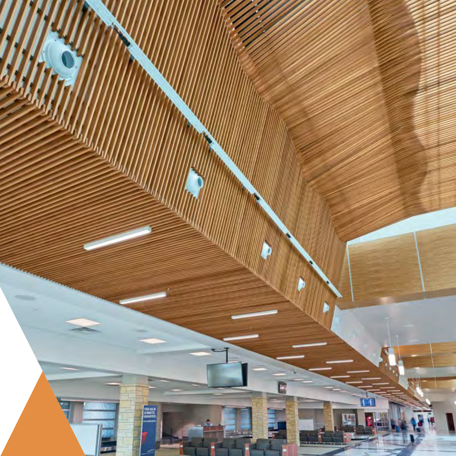
▲ WoodWorks® Grille; The Eastern Iowa Airport, Cedar Rapids, IA; Mead & Hunt, Inc., Minneapolis, MN
