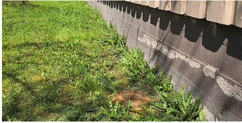
Foundation - Before ElaProof™
