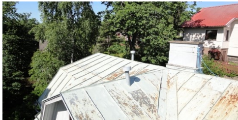
Tin roof - Before ElaProof™
