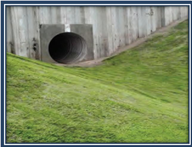
**Figure 76. Example of the use of hydro-turf ([www.acfenvironmental.com](http://www.acfenvironmental.com))**
