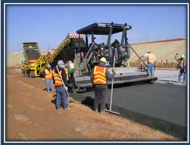
**Figure 75. Laying Roller Compacted Concrete ([www.theconstruction.org](http://www.theconstruction.org))**
