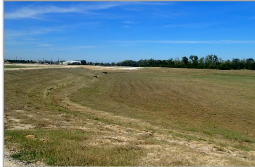
**Dry-Bottom Basin:** Includes pilot channels and cross slopes to facilitate mowing and complete drainage of a basin following a storm event.
