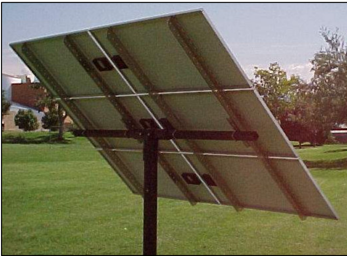
Mounts on Schedule 40 Steel Pipe
