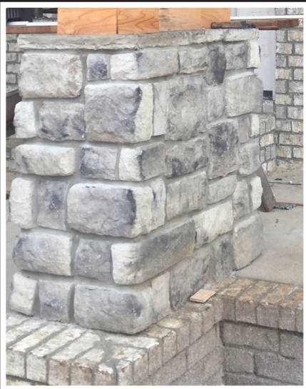
METRO GREY RUBBLE WITH GROUT JOINT SHOWN ON COLUMN BASE
