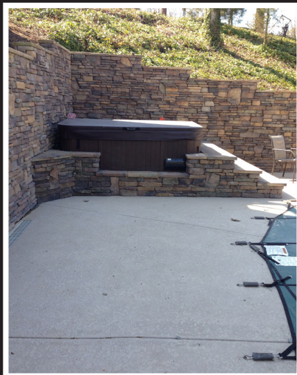
ASPEN STACK. RETAINING WALLS, STEPS, PORCH SURROUND
