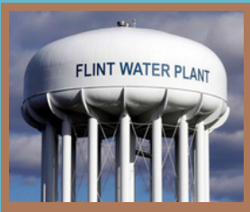
Flint Water Plant
