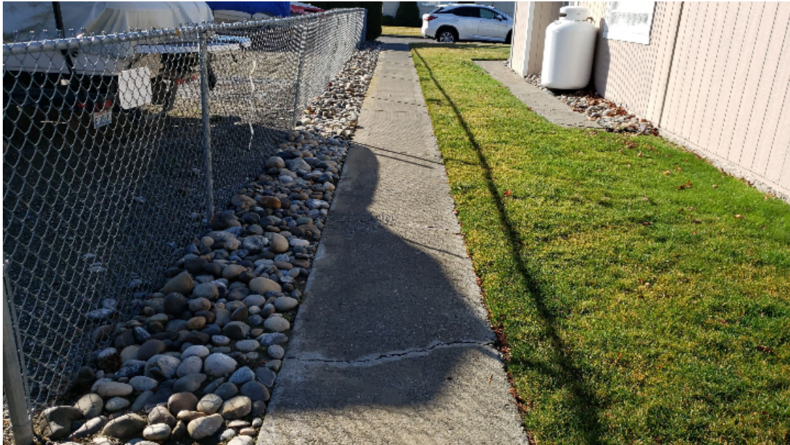
General Site - Concrete, Sidewalk, 10% Replace
