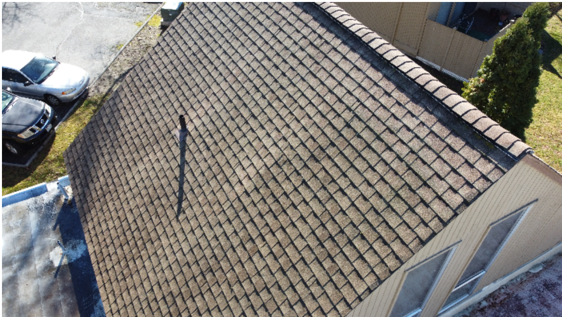
Building Exterior - Roof, Asphalt Shingle
