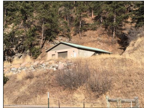
Figure 9. Turkey Creek Treatment Plant.
