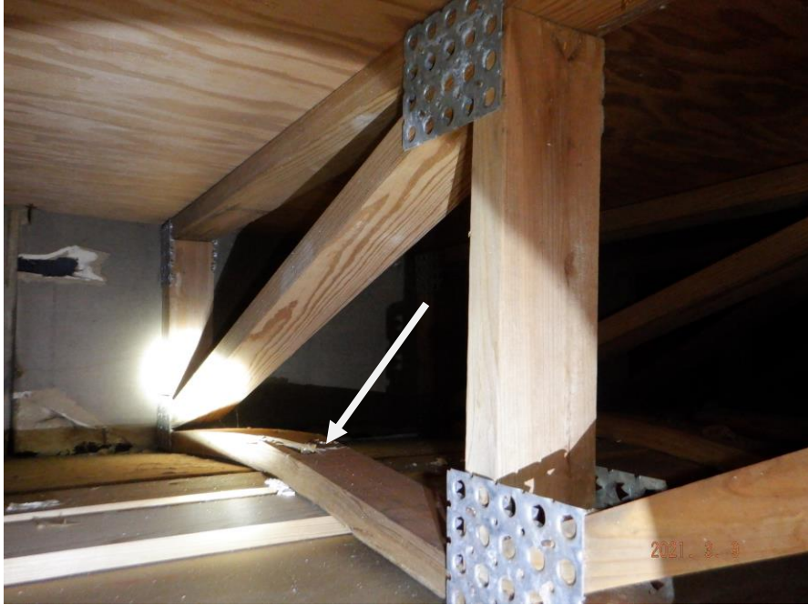
Photo A, Typical Bottom Chord Truss Damage
