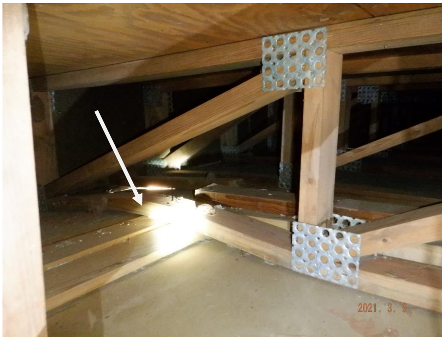
Photo B, Typical Bottom Chord Truss Damage
