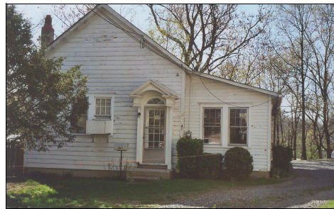
Club Apartment prior to the Spring 2003 re-siding
