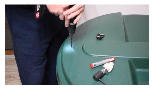
Make the hole larger using the special drill bit.
