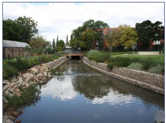
Example of Gabion Wall
