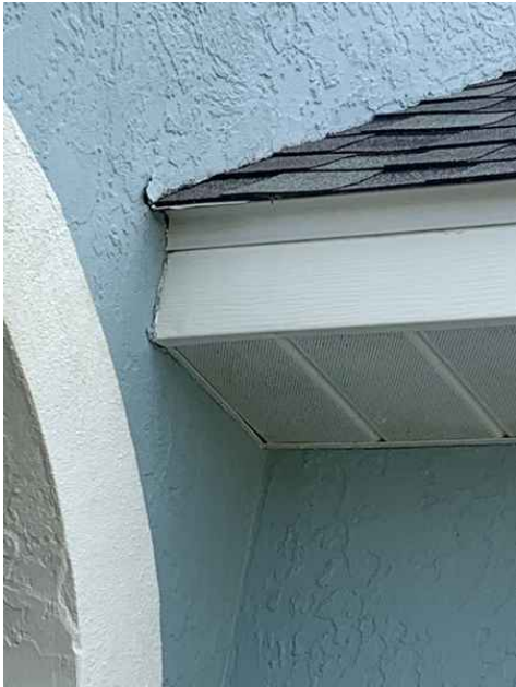
Missing Kickout
