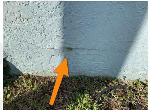
Crack with vegetation
