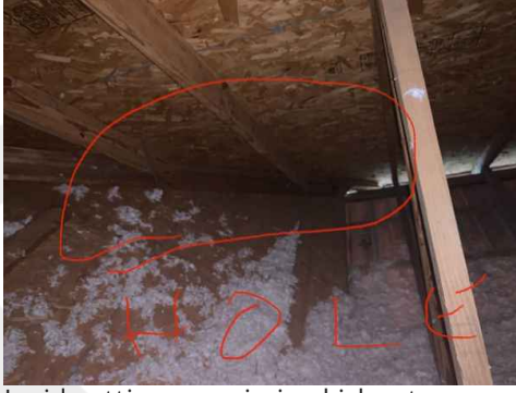
Inside attic near missing kickout
