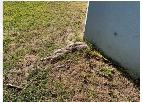
Roots growing into foundation Southeast corner
