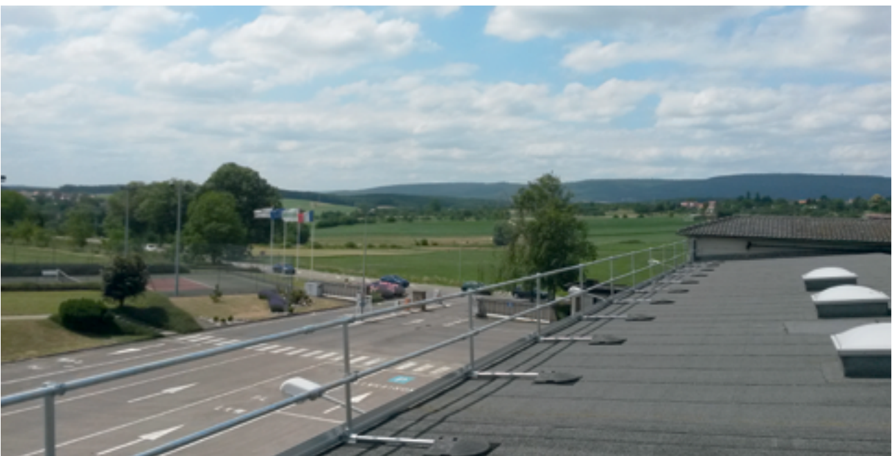
Figure 17 Temporary flat-roof edge protection (image courtesy of Safesite Limited)
