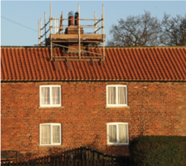
Figure 24 A traditional chimney scaffold
