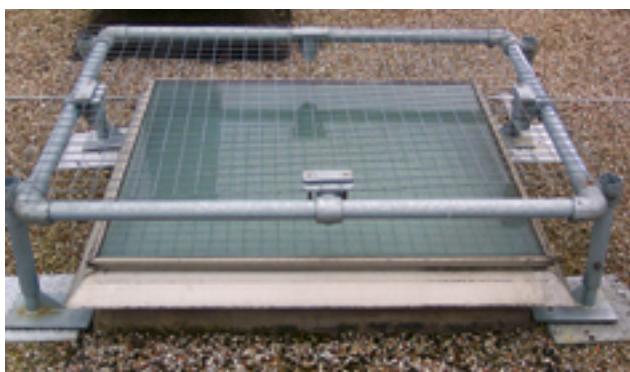
Figure 43 Covers can be fitted to existing roofs or included as part of the design (image courtesy of Safesite Limited)
