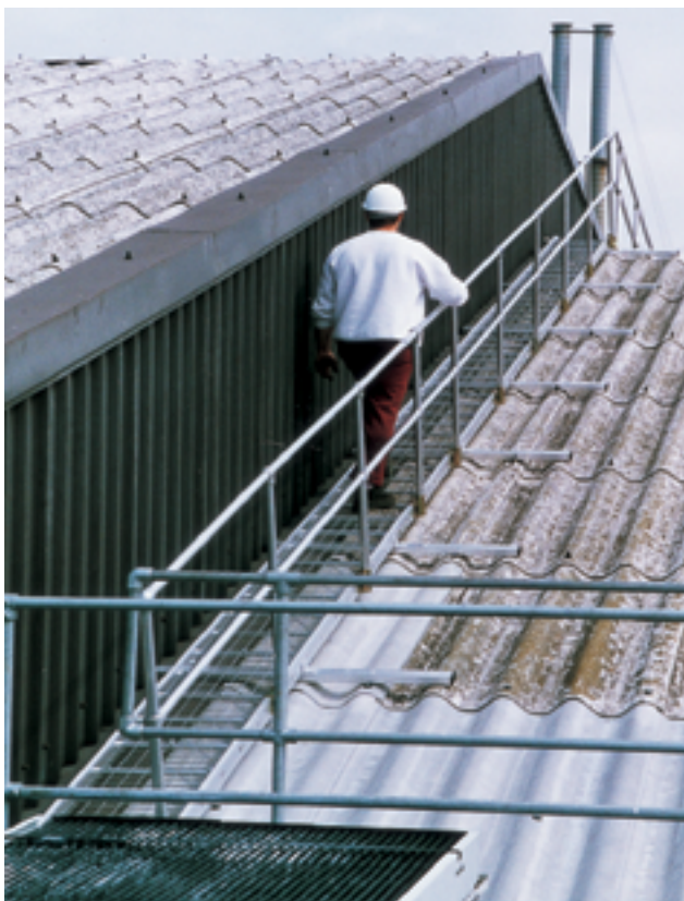
Figure 37 (left) Permanent walkway giving safe access on a fragile roof (this walkway was retrofitted, but similar access can be included in initial designs)
