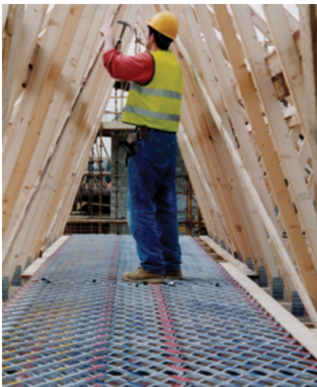
Figure 14(a) Decking system that provides a working platform in the roof eaves (image courtesy of Oxford Safety Components Ltd)
