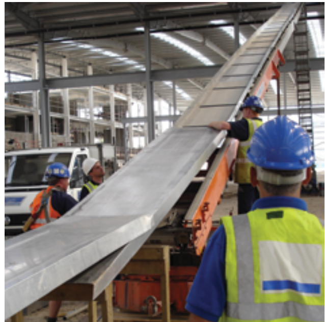
Figure 35(a)–(c) Mechanical handling of large roof sheets (images courtesy of Advisory Committee on Roof Safety)
