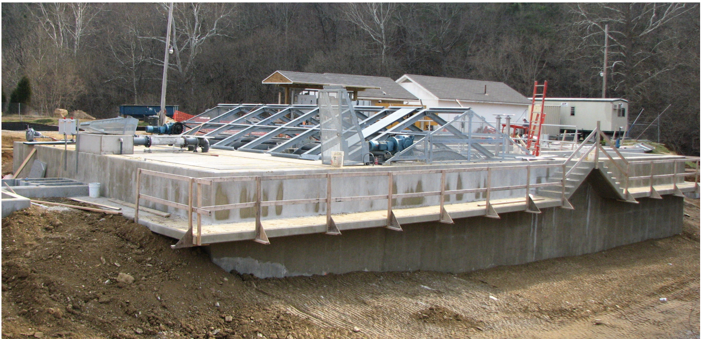
Fincastle Wastewater Treatment Plant while under construction
