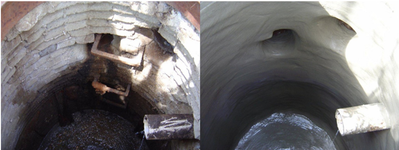
Same Manhole Before and After Rehabilitation
