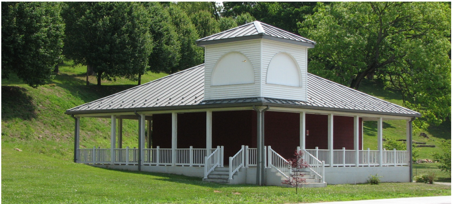
Park Avenue Well Exterior Chlorine Contact Tank Encircles Building under the Wrap-Around Porch
