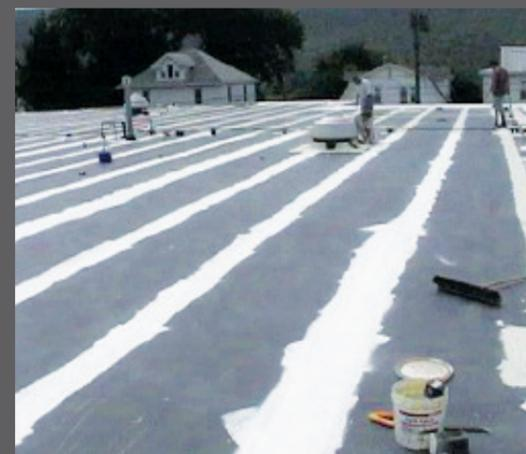
After proper cleaning and application of appropriate primer, Spunflex® is embedded into the base coat, over the seams, and at penetrations.
