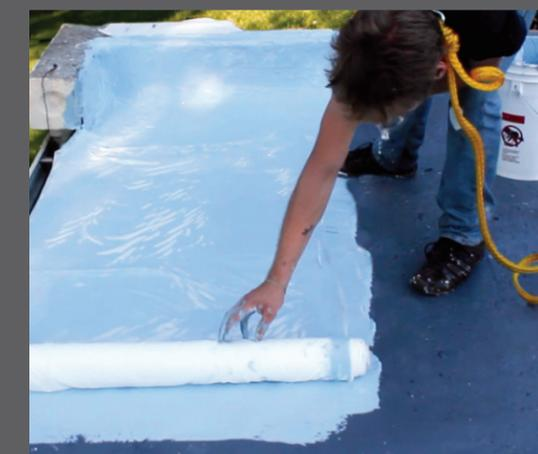
Fabric is embedded into another layer of base coat, then applied in overlapping sheets over the entire roof to form a seamless, monolithic surface.
