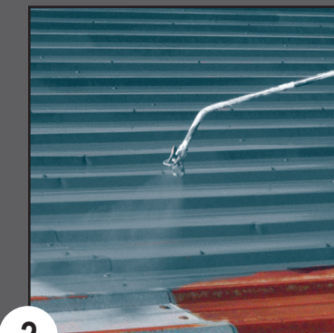
2 Prime with Conklin Encase® Metal Primer.
