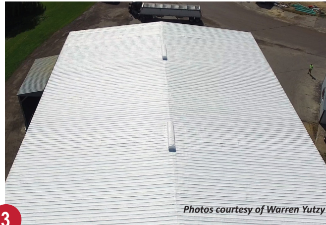
Metal roof after Benchmark® acrylic top coat.
