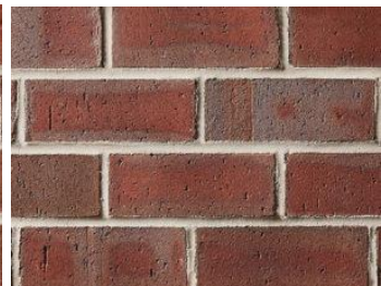
Town Hall Brick
