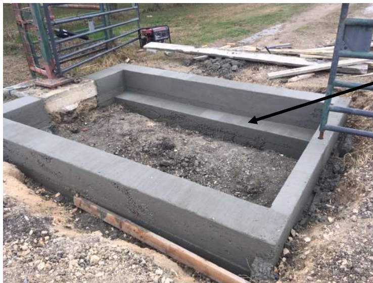
Figure 3 – Concrete Foundation including Footing
