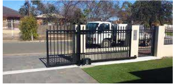
Gates on tracks
