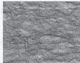
CSP 6 (heavy shotblast)
