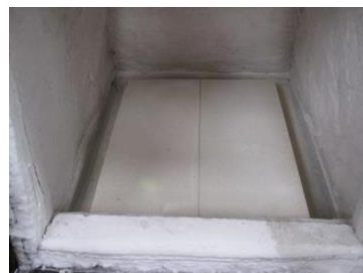
Both base shelves in place
