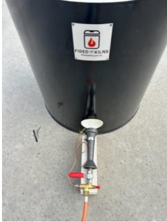
Above Image shows correct burner positioning
