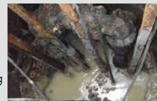
FOG and sludge accumulation blocking equipment (top) H 2 S corrosion & FOG (above)
