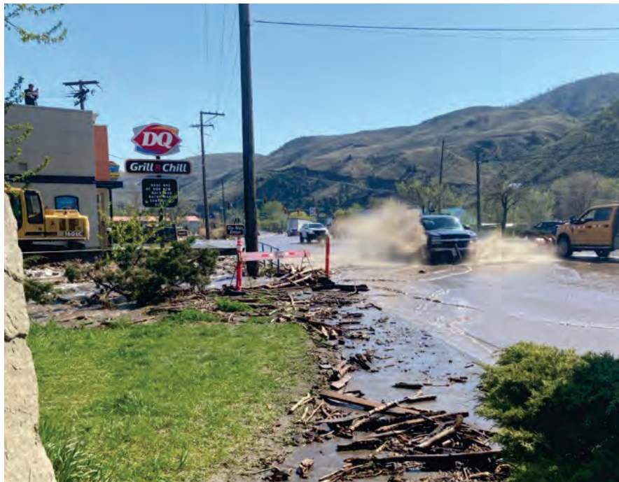
FIGURE 1-1: CACHE CREEK FLOOD WATERS ON HIGHWAY 97 (MAY 03, 2023)
