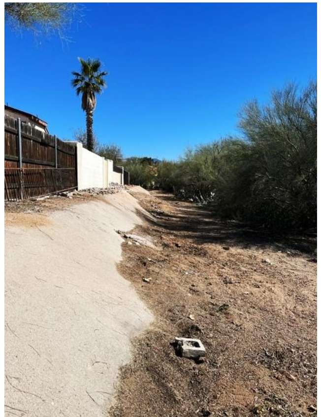
(Doria bridge East side) ...After
