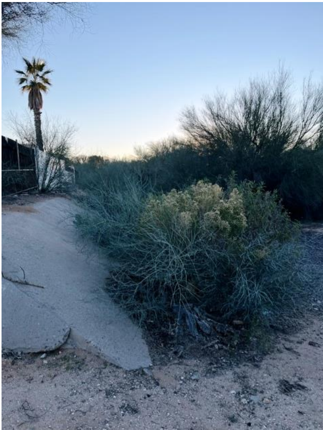
(Doria bridge East side) Before
