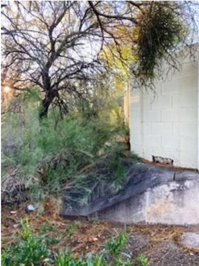
(Doria East side of alley) Before
