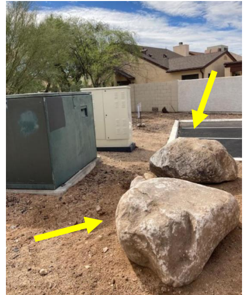
Boulders placed around front and side of electric transformer where vehicle jumped curb back on 5-28-22.
