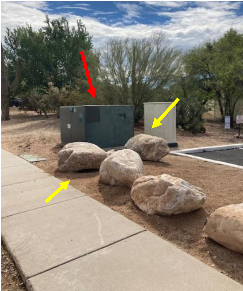
Electric Transformer box (red arrow)
