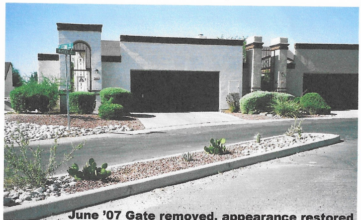
June '07 Gate removed, appearance restored
