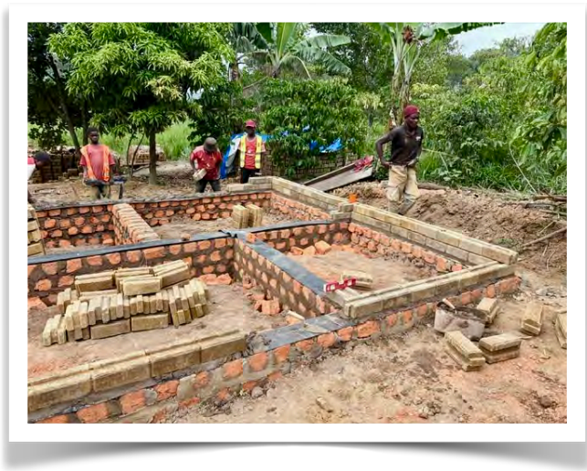
New design of locking brick house that Alan and Jeanne helped to build.
