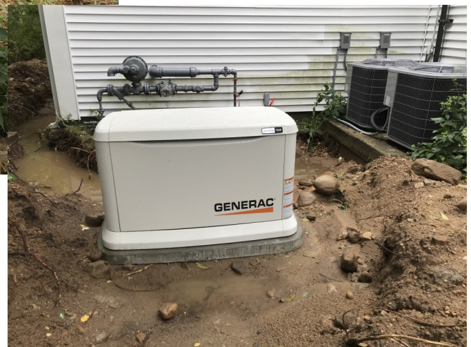
The generator on 9/16 with the protective shroud installed.
