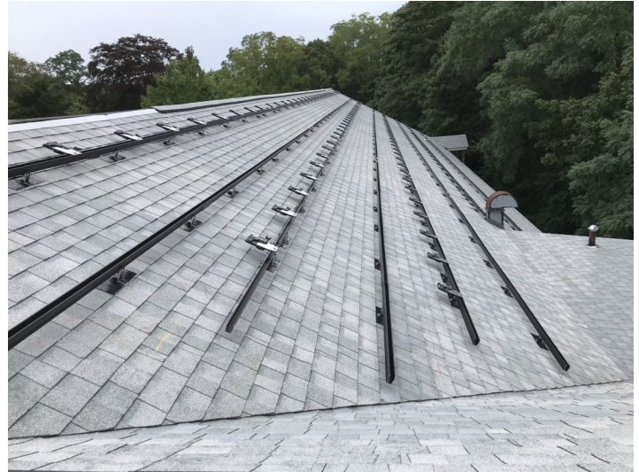
The rack system that holds the PV panels on Fellowship Hall roof.
