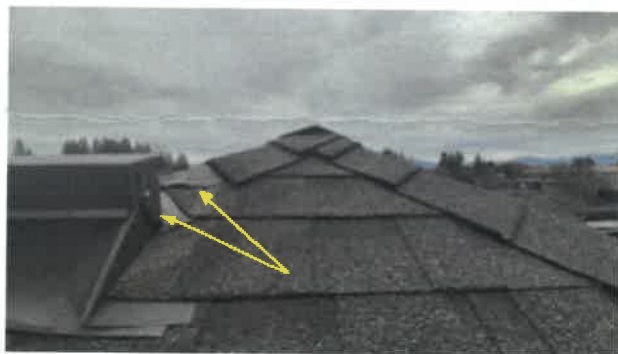
9 Shows 2 exposed common fasteners at the South facing roof area
