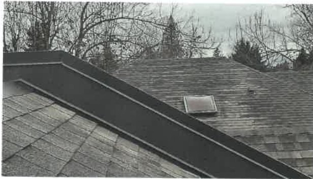
5 Shows the separation/Firewall metal flashing details in good condition and well fastened
