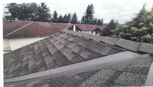
15 An overview of the West facing roof area. The shingles and ridge cap shingles are in good condition throughout
