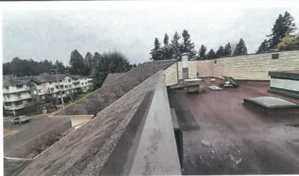
13 An overview of the metal cap flashings
