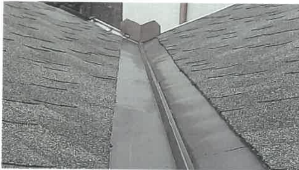
7 Shows the metal valleys in good condition being clear of debris
