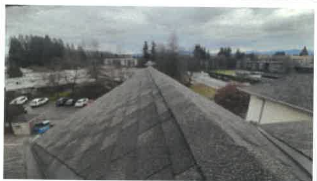
8 Shows the ridge cap shingles in good condition and well fastened
