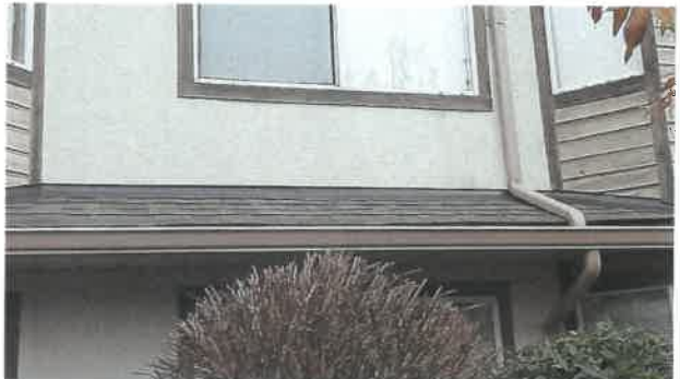
20 The metal transition wall flashings are in good condition and well fastened throughout the lower area
