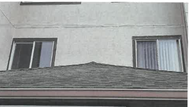
21 The shingles and ridge cap shingles are in good condition and well fastened throughout the lower roof area
