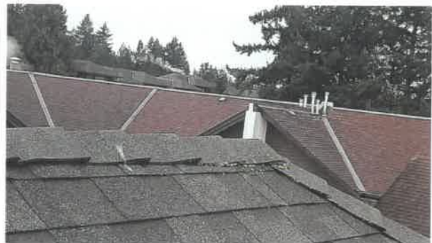
18 Shows a minor area of organic growth(moss) at the ridge of the NW corner area
