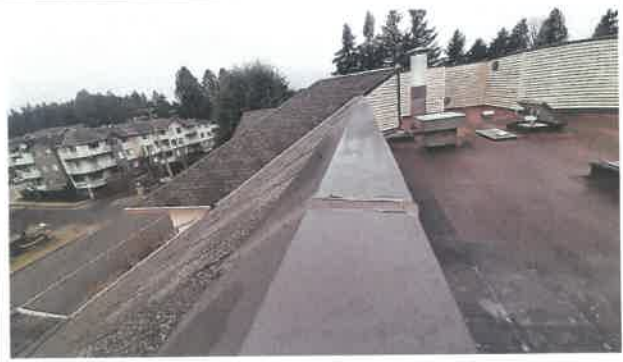
14 The metal cap flashings are in good condition, being well fastened and the sealants in good condition and sealed. This is typical throughout the roof area
