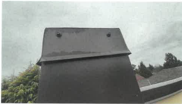
17 A closer view showing the metal cap flashings in good condition and well fastened with the fasteners properly driven and seated
