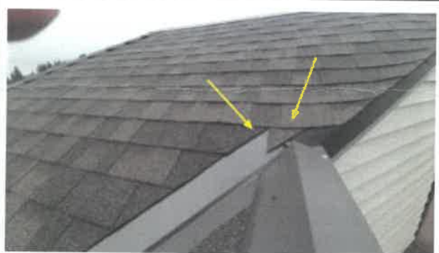
10 Shows an exposed common fastener in the valley and a shingle that has slipped
