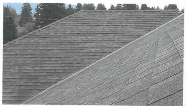
6 The shingles are in good condition and well fastened throughout the area
