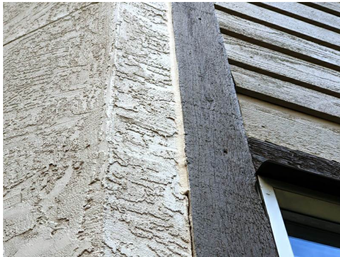
Photo No. 7: Joint sealants
