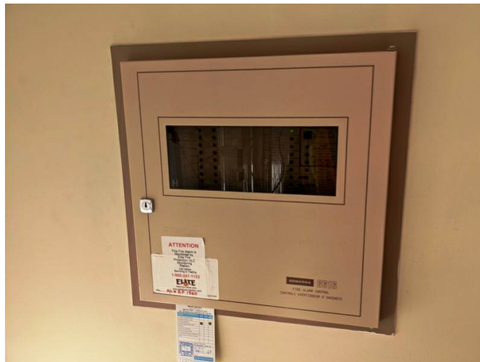
Photo No. 13: Fire alarm panel
