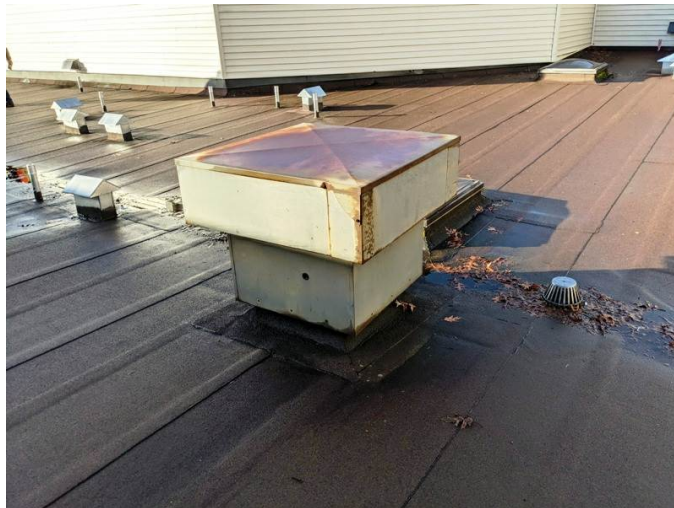
Photo No. 22: Make-up air unit
