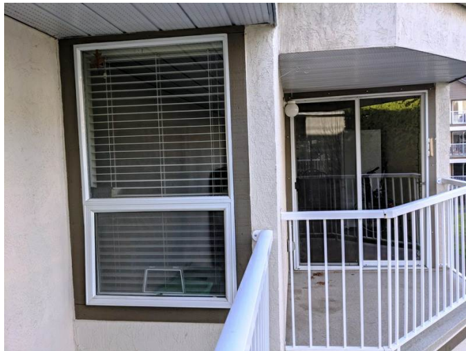
Photo No. 10: Aluminum-framed window and sliding door
