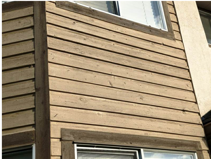
Photo No. 6: Wood cladding and trims
