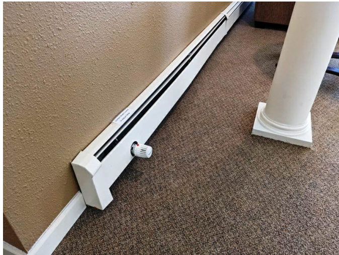
Photo No. 21: Hydronic baseboard heating
