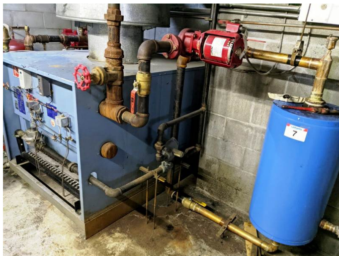
Photo No. 20: Hot water boiler and heat exchanger
