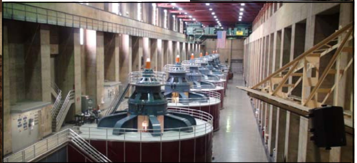
Power Generators in Hoover Dam
