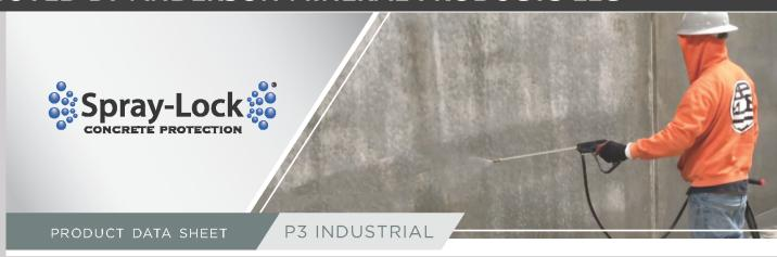
P3 Industrial is a spray-applied product which uses Spray-Lock Concrete Protection (SCP) colloidal silica technology to provide a permanent increase in the durability and lifespan of Portland cement concrete.
