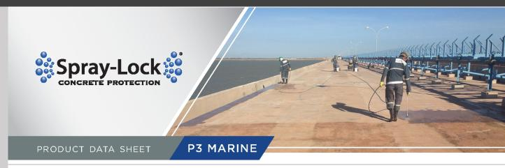
**P3 Marine** is a spray-applied product, based on Spray-Lock Concrete Protection (SCP) colloidal silica technology, which provides a permanent improvement that increases the durability and life cycle of Portland cement concrete.
