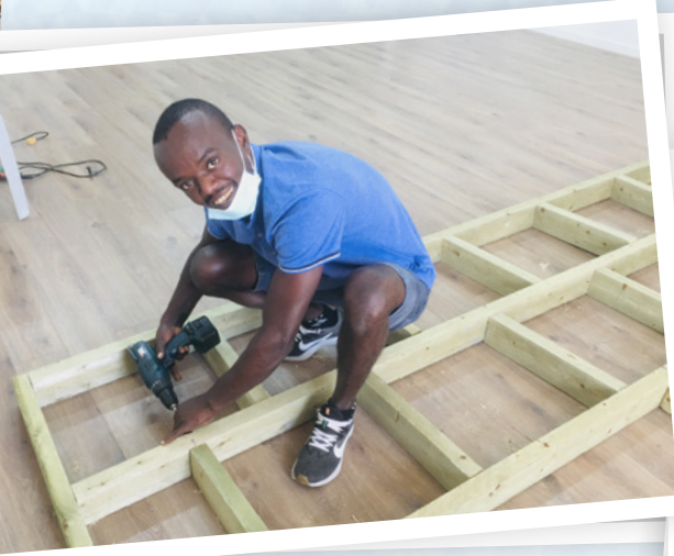
Stefanos building the stage in Beresheet's newest meeting place
