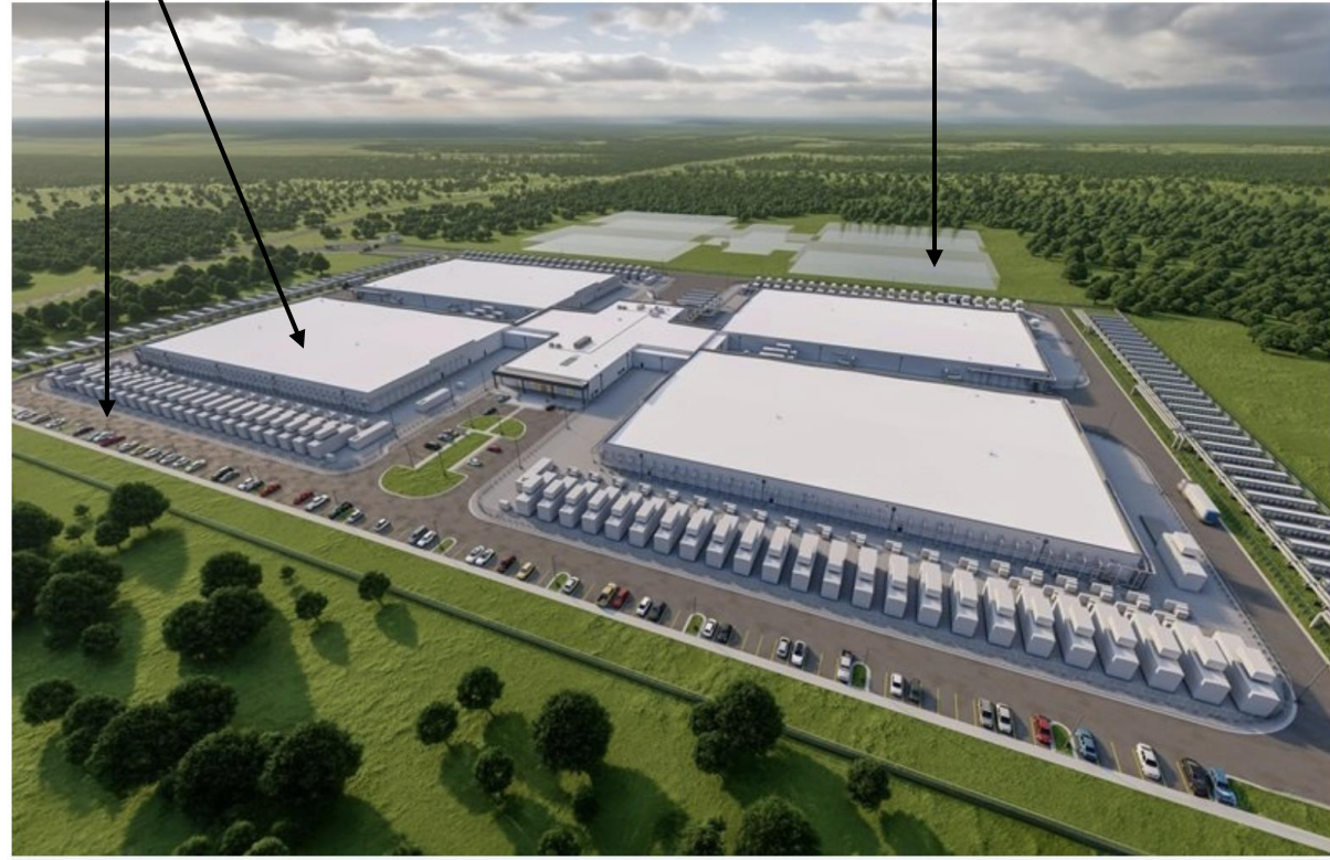
The Lancium Clean Tech data center campus is being constructed by contractor DPR Construction in Abilene, Texas, with Crusoe Energy as its developer.
