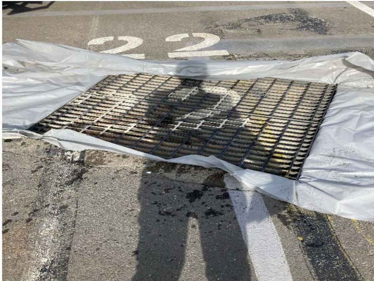
Caption: Storm drain sampling - Space K22, 8/14/2023, Port of Oakland.
