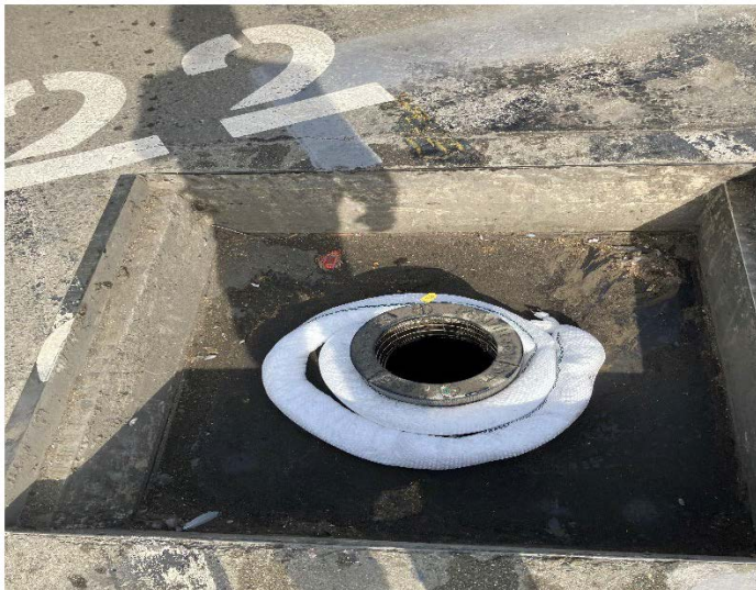
Caption: Storm drain sampling- Space K22- Open, 8/14/2023, Port of Oakland.
