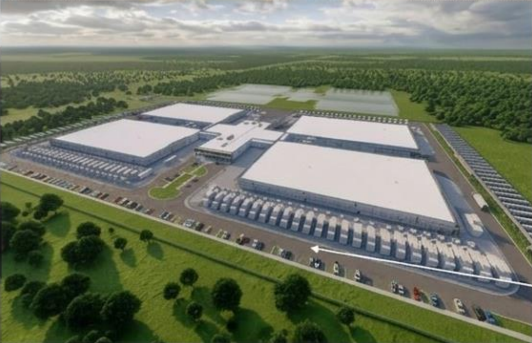
The Lancium Clean Tech data center campus is being constructed by contractor DFR Construction in Abilene, Texas.
