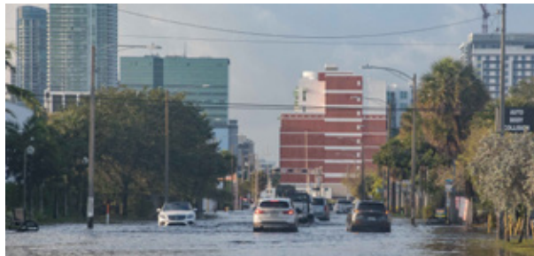
Storm floods in downtown Fort Lauderdale, 2023.
