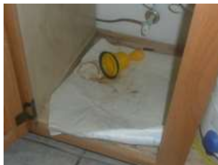
2) The kitchen cabinet under shelf has been water damaged
