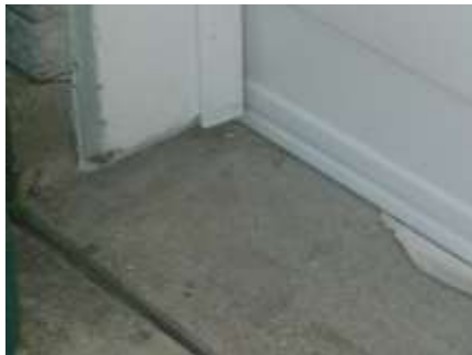
The weather stripping at the garage is torn
