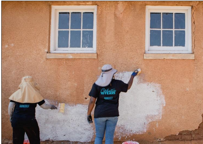
Lime Wash Being Applied
