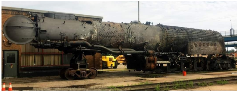
Big Boy Boiler
