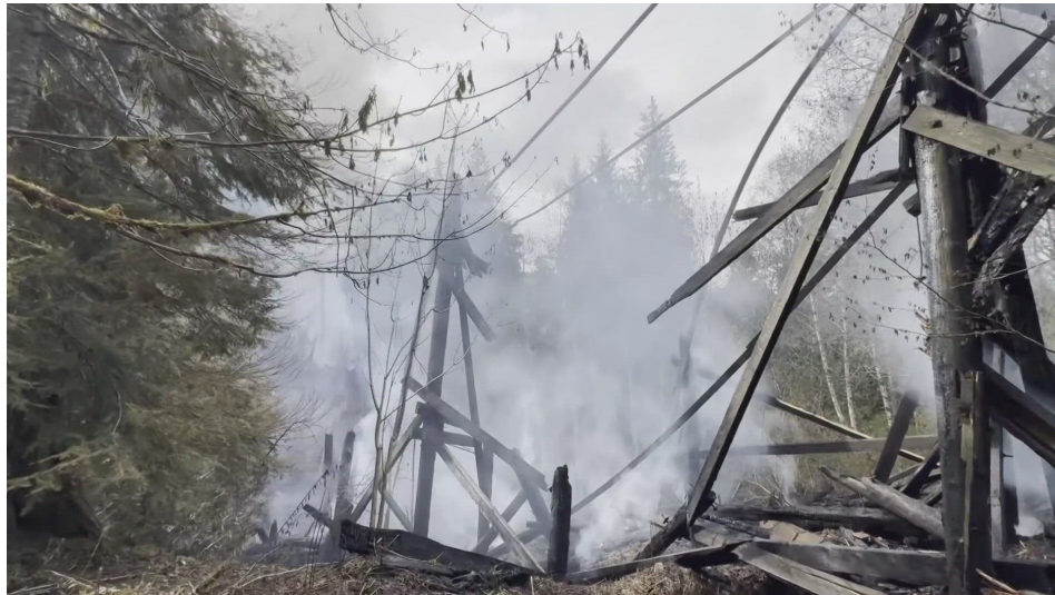
Collapsed railroad trestle, still smoldering.
