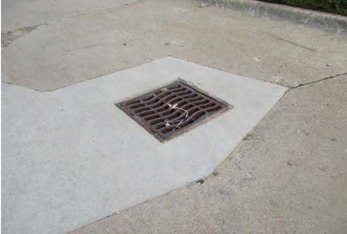
Overview of a previously repaired catch basin
