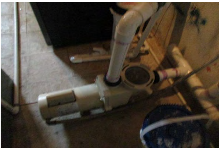
Overview of the 2-hp pump for the pool
