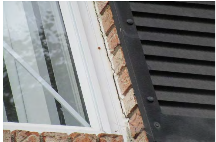
Isolated condition of a crack in the sealant of a window jamb
