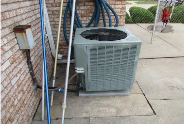
Overview of the 5-ton condensing unit for the clubhouse
