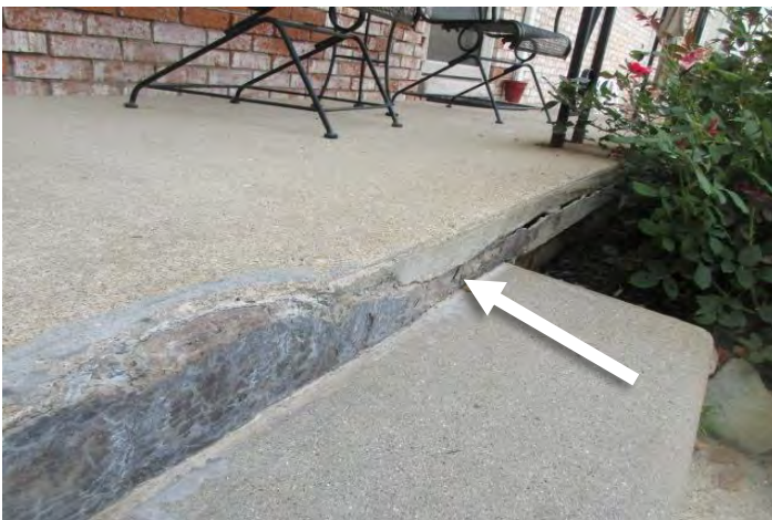
Isolated condition of a damaged entry stoop
