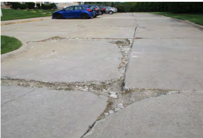
Isolated condition of significant damage to a concrete street
