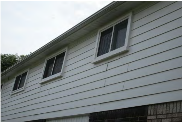
Some sided surfaces are aluminum siding, as seen in this photo
