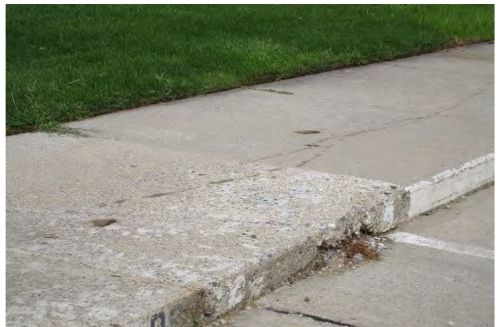
Isolated condition of surface spalling at a portion of sidewalk
