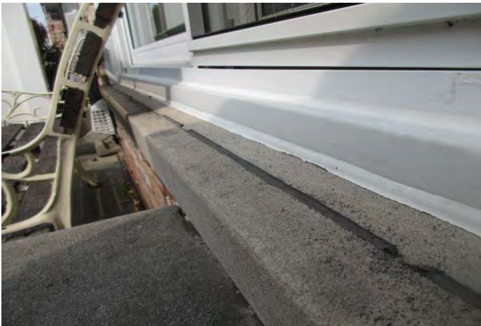
Overview of typical sealant at a window sill
