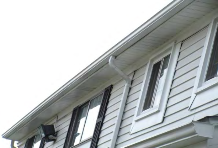
Overview of a typical soffit and fascia
