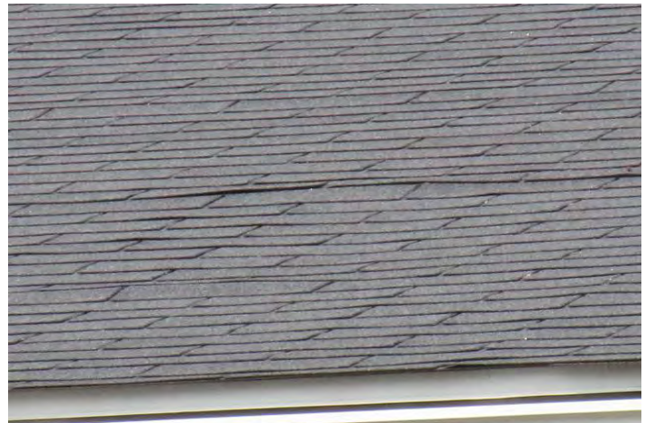
Isolated condition of shingles that have some "lift"
