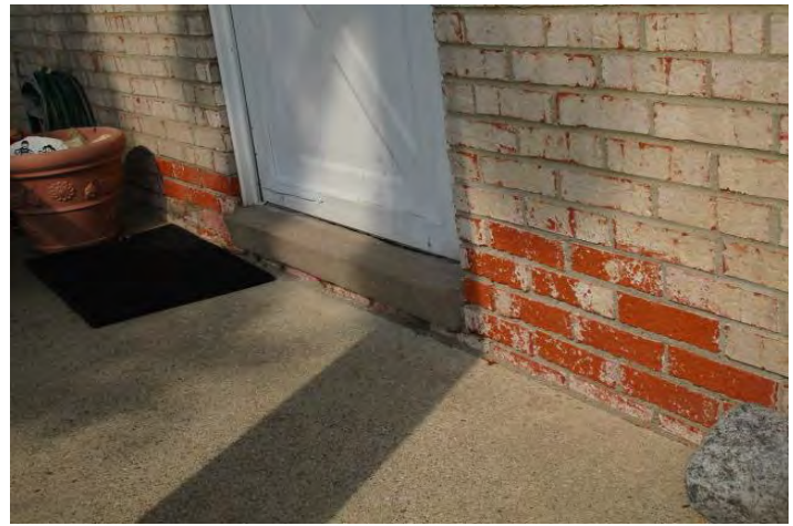
Overview of spalled faces at masonry bricks
