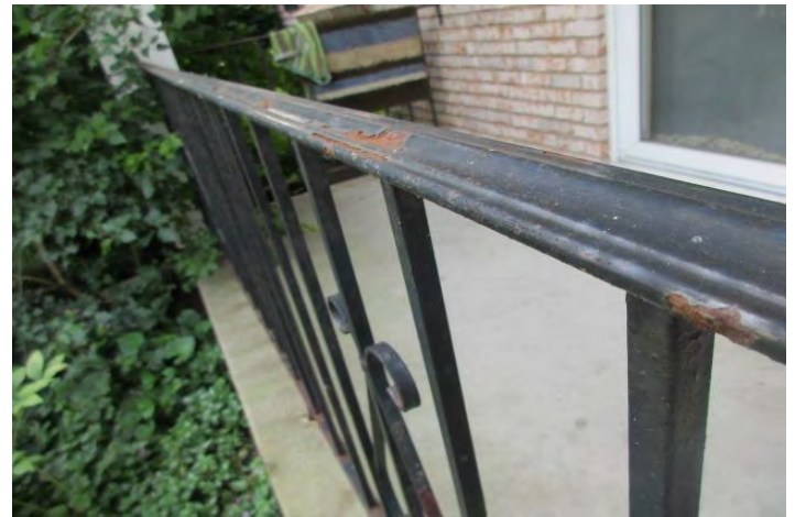
Example of chipped paint and metal oxidation at a top rail
