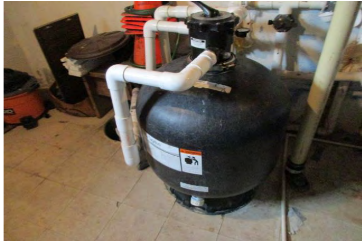
Overview of the sand filter for the pool
