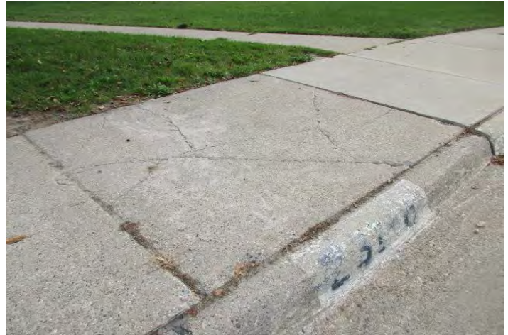
Isolated condition of cracks in a section of sidewalk
