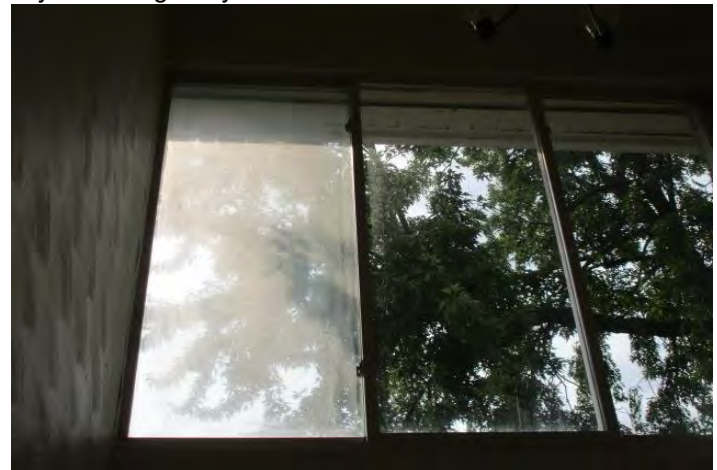
Isolated condition of a common area window that has a broken seal
