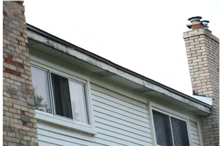
Isolated condition of missing gutter and fascia
