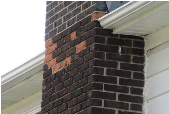
Overview of spalled faces at masonry bricks
