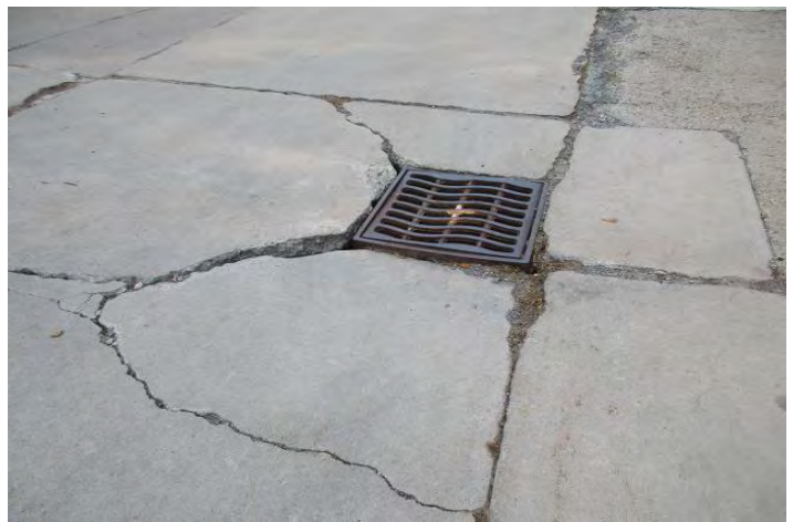
Isolated condition of damaged concrete around a catch basin
