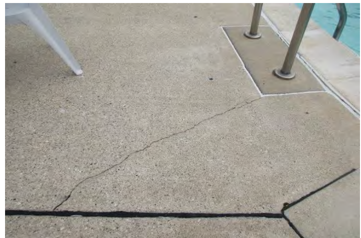
Isolated condition of a crack in the concrete deck
