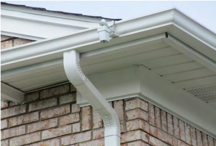
Typical gutter to downspout connection
