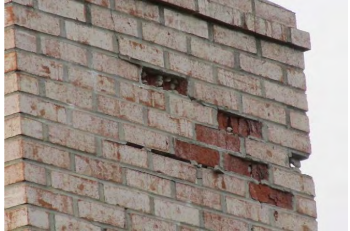
Overview of spalled faces and damage at masonry bricks
